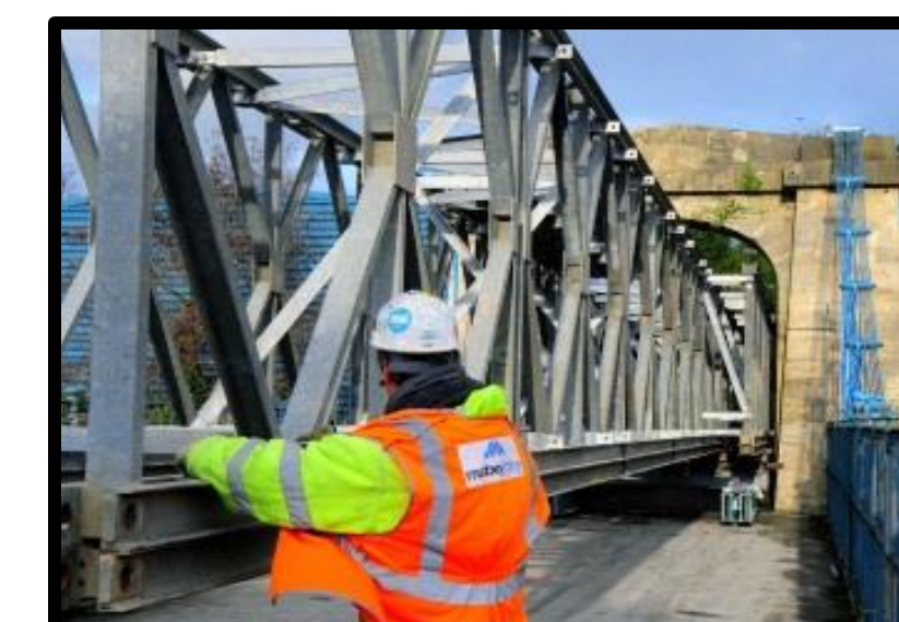
Figure 5: Maintenances work going on
