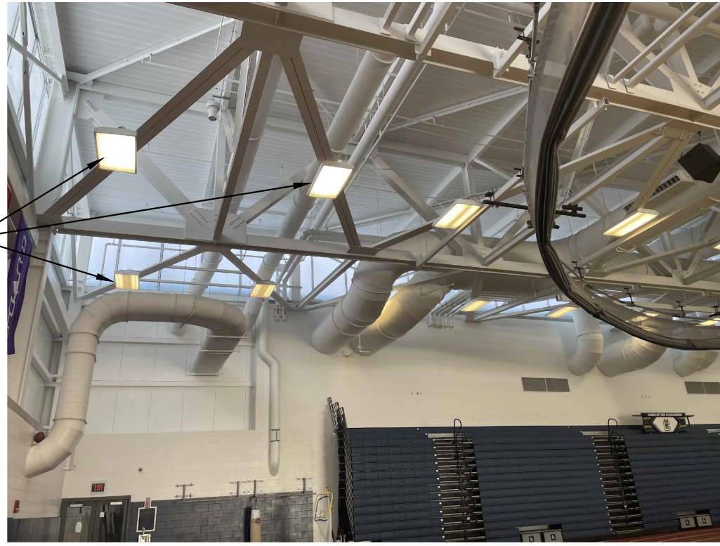
1 PHOTO OF EXISTING FIELDHOUSE LIGHT FIXTURE SCALE: N/A
